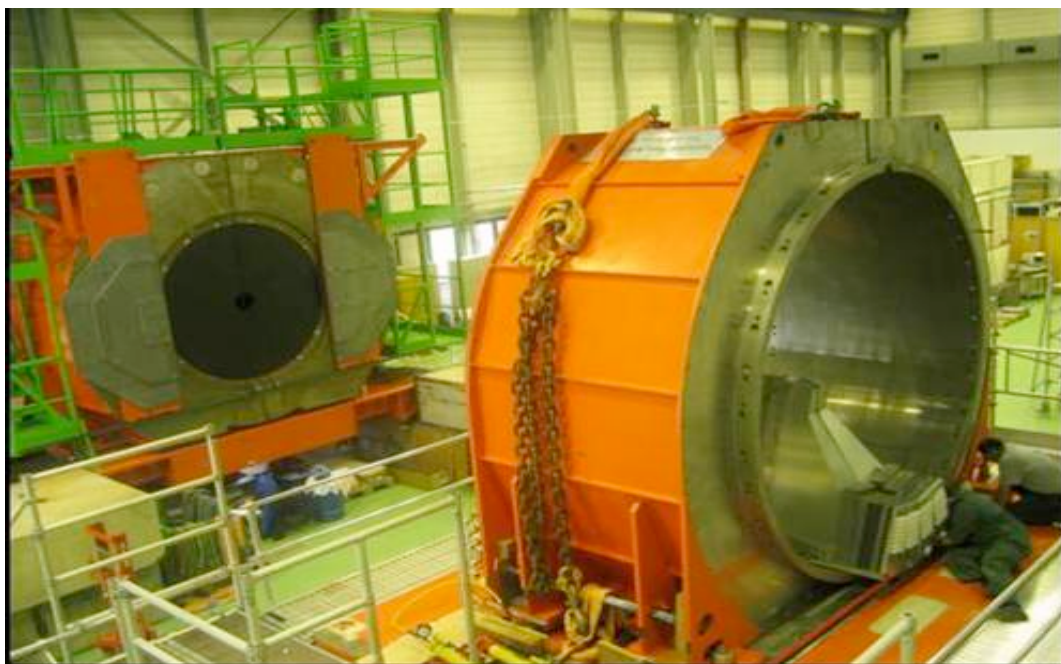
Figure CP 10: Assembled HF modules in building 186 at CERN.
